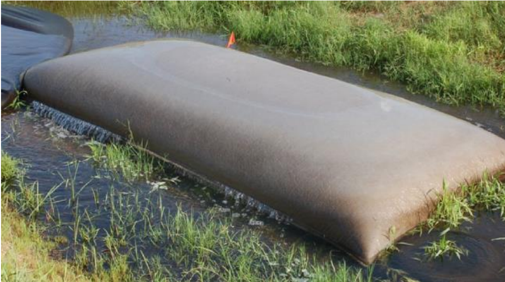
Figure 30 - Silt Bag Filtering
