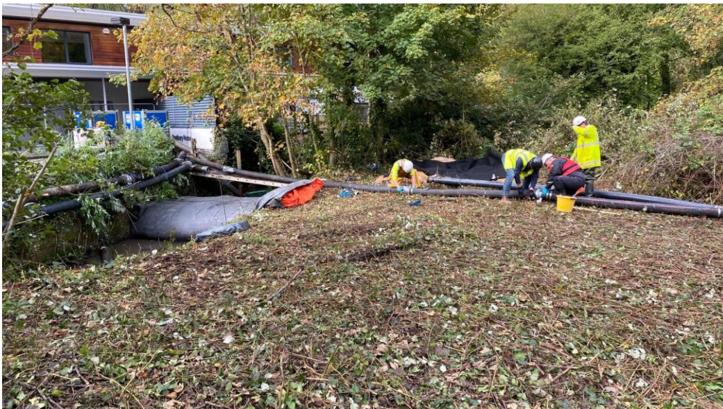
Figure 12 - Water Filled Dam - River Itchen
