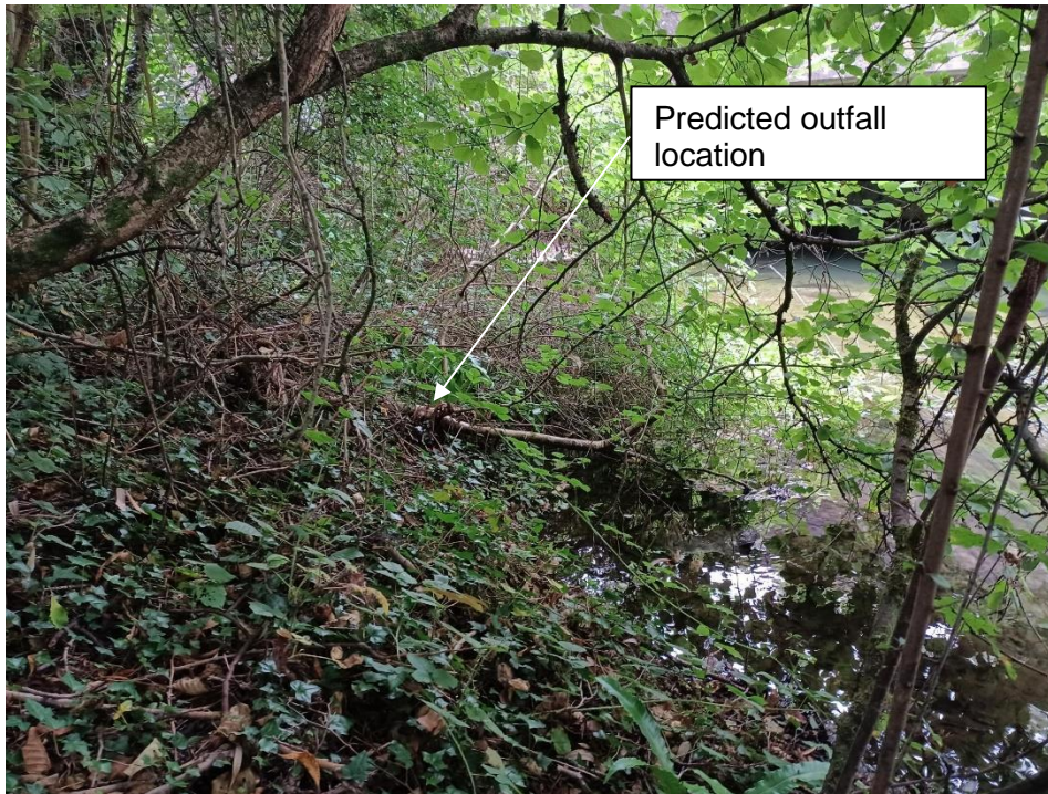
Figure 32 - Heavily Vegetated Area Over Existing Outfall
