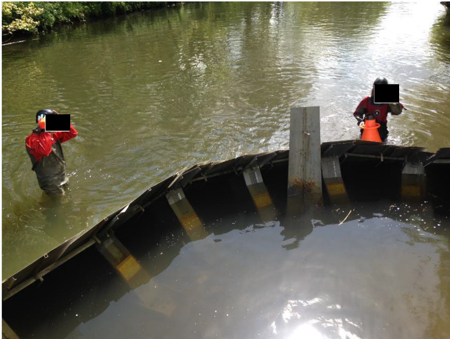
Figure 7 - Steel Sheet Facing
