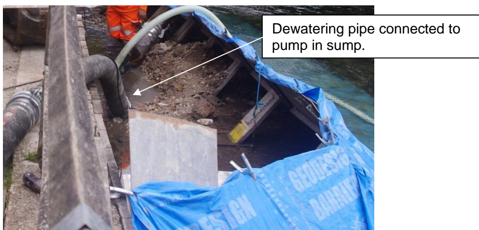
Figure 26 - Dewatering in River Itchen
