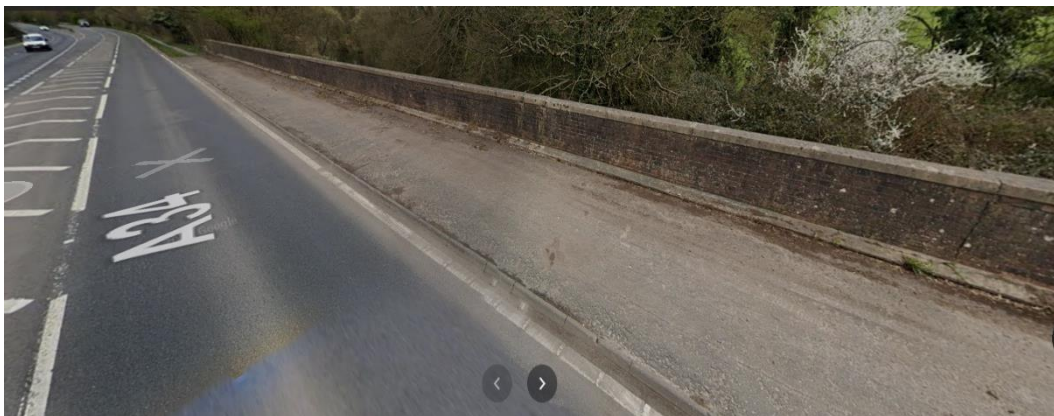
Figure 35 - Kings Worthy Bridge Hardstanding / Footpath
