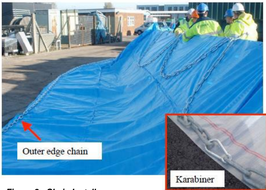
Figure 8 - Chain Install
