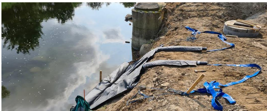
Figure 13 - Positioning of Deflated Dam
