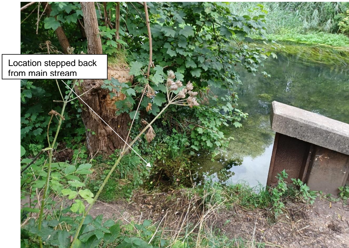
Figure 43 - Outfall 3 Location Stepped Back
