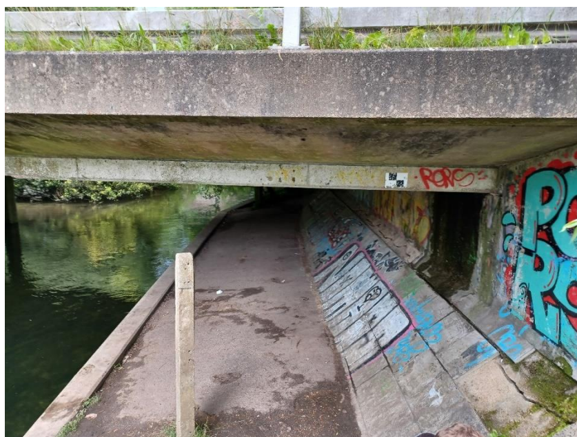
Figure 44 - PRow Underneath Itchen Bridge
