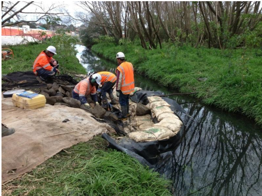
Figure 22 - Dewatered Working Area
