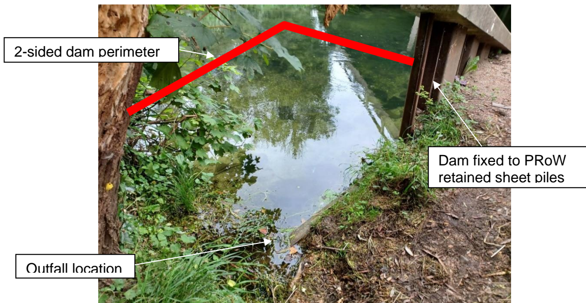
Figure 45 - Outfall 3 Isolation Configuration 1
