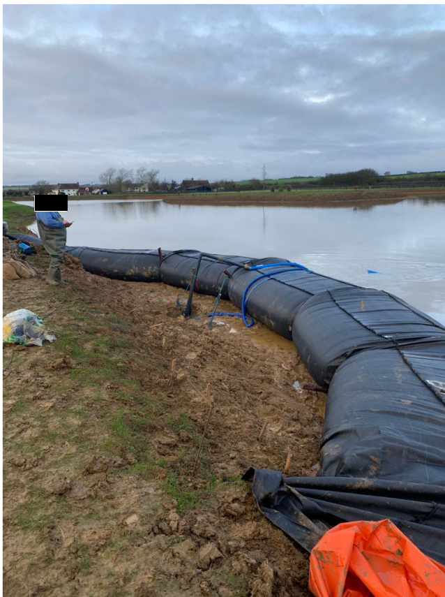
Figure 15 - Dewatered Working Area
