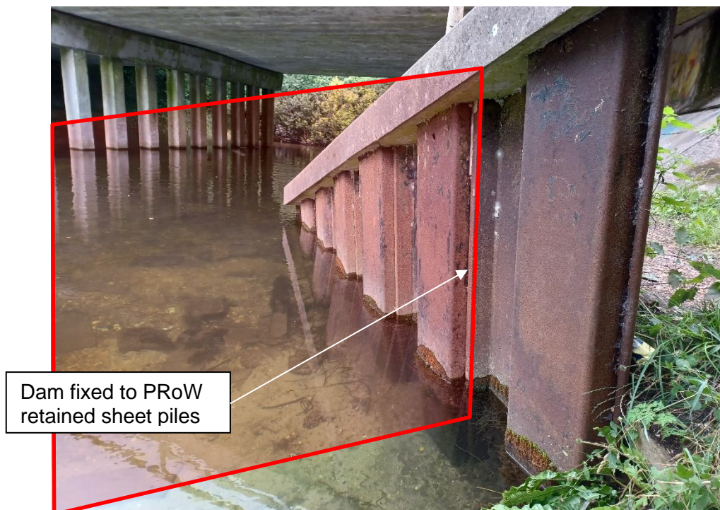
Figure 47 - Outfall 3 Isolation Configuration 3
