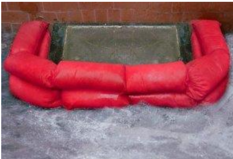
Figure 20 - Polythene Sealed Sandbags
