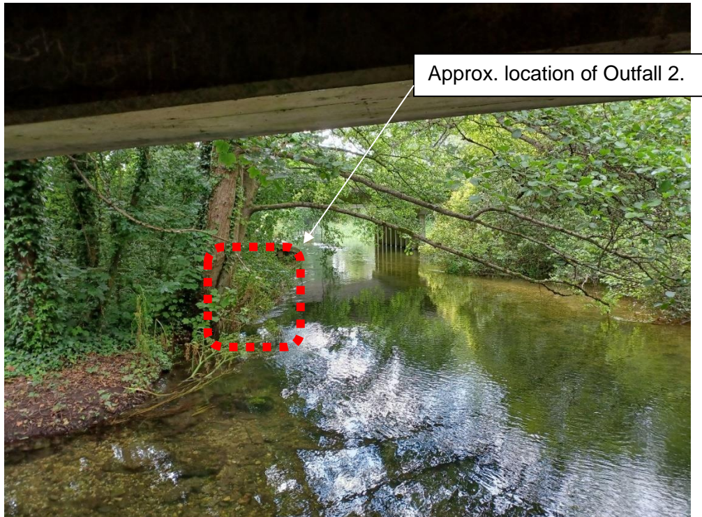
Figure 38 - Outfall 2 View from Kings Worthy Bridge
