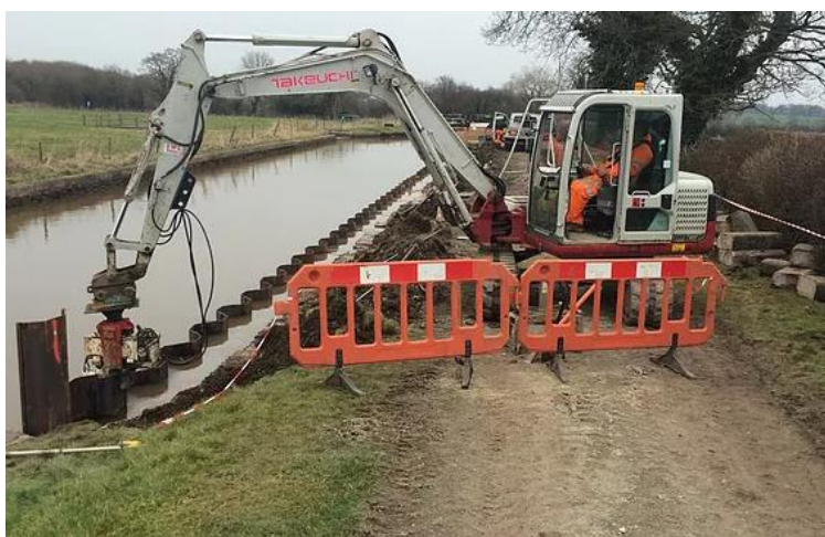
Figure 23 - Machine Attached Piling Hammer
