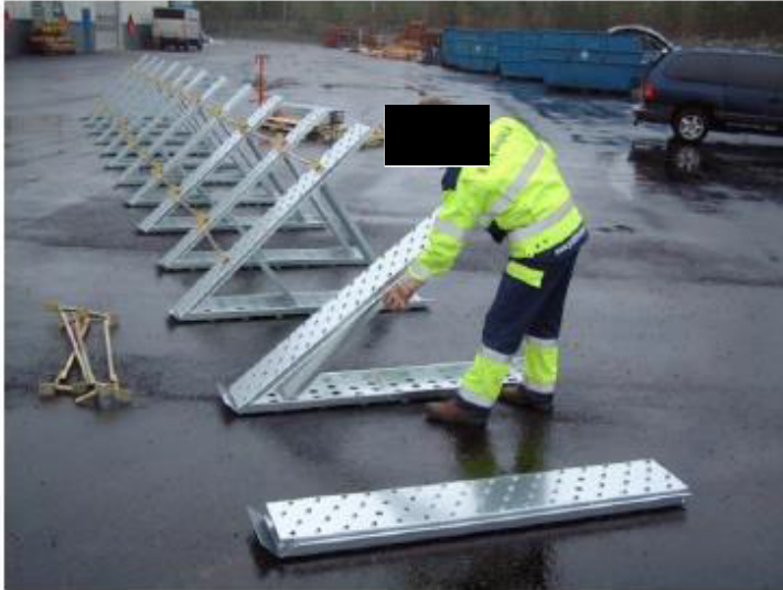
Figure 5 - A-frame Assembly
