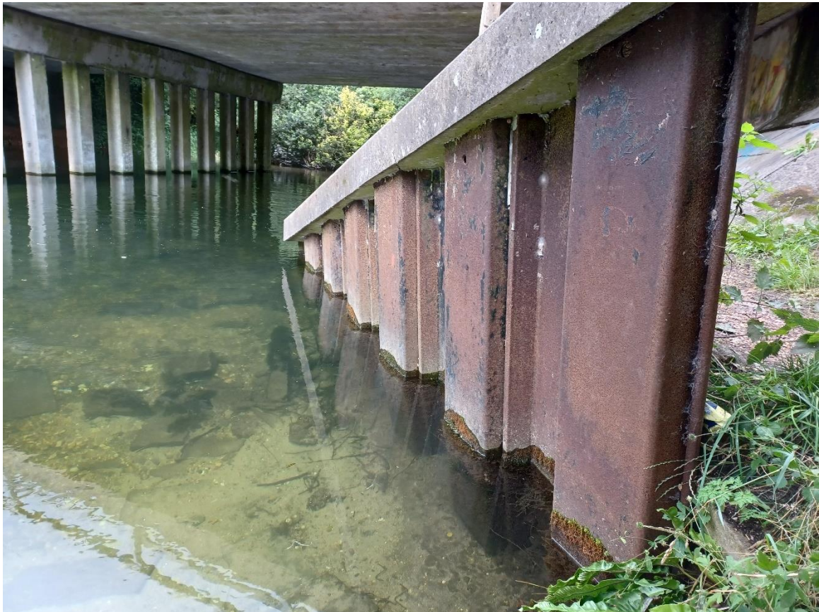
Figure 42 - PRow Sheet Pile Retaining Structure
