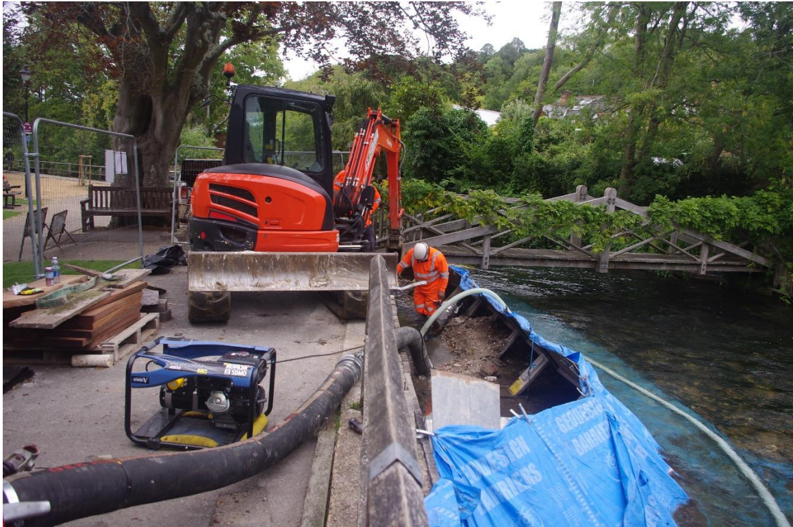
Figure 3 - River Itchen Central Winchester Framed Dam
