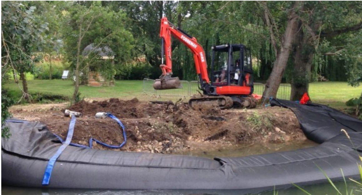
Figure 9 - Water Filled Dam
